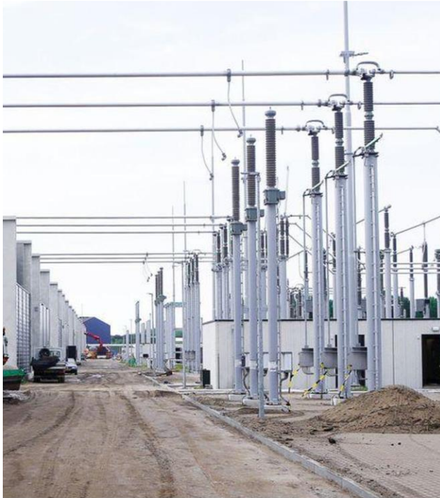
Expand in grids and EV charging
