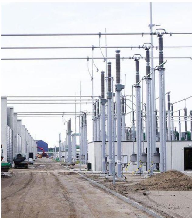
Expand in grids and EV charging
