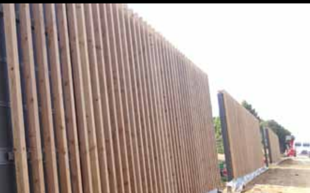
Betonac. Lummen acoustic barriers.
