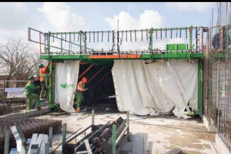
BAM Materieel. Patented tunnel lining for residential projects.
