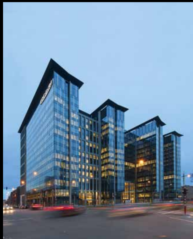
Interbuild. North Light and Pole Star office blocks, Brussels.
