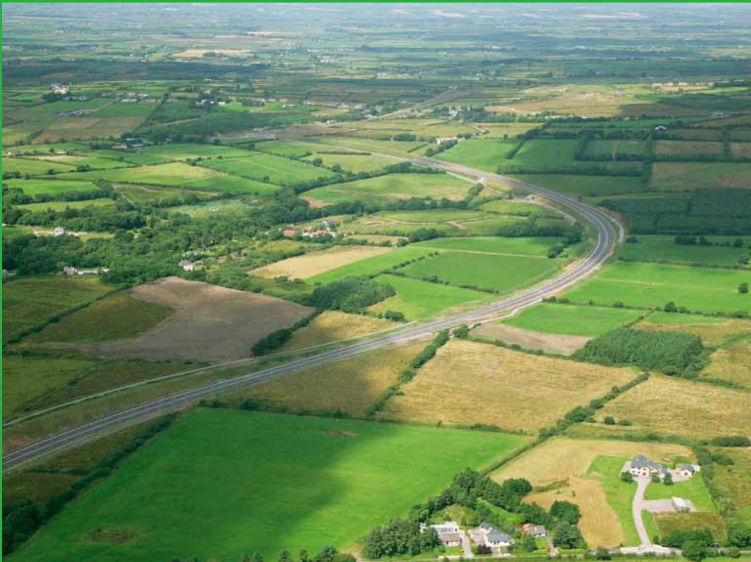
BAM Contractors. 13.5 kilometre long N22/N69 bypass around Tralee, Ireland.
