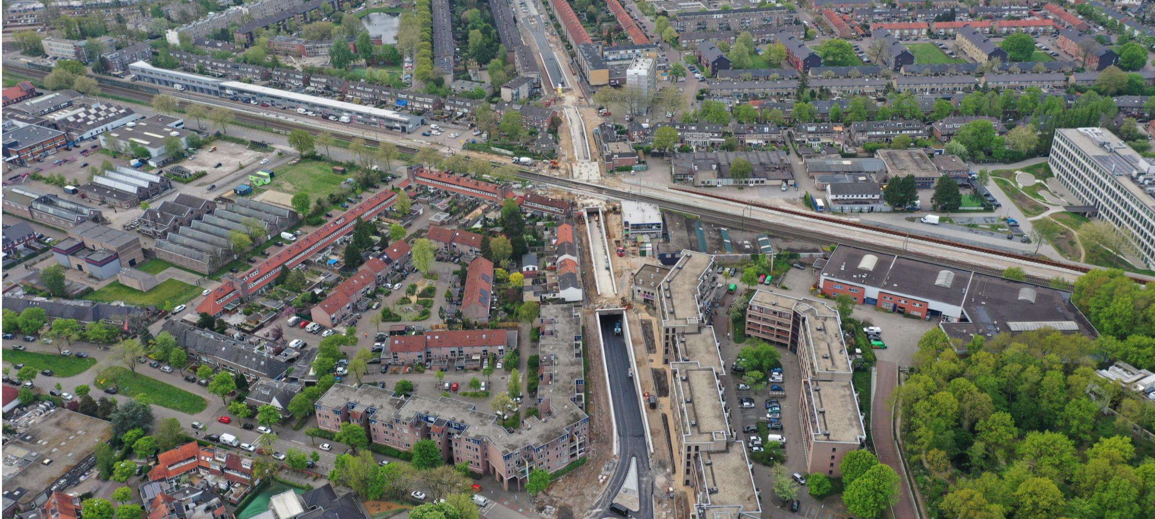
Alexiatunnel (249 metres), Hilversum, crossing railway line Hilversum - Amersfoort and the HOV track Hilversum - Huizen. The tunnel has two tubes above the other: the lower for motorised traffic, the upper for cyclists and pedestrians – BAM Infra Nederland
