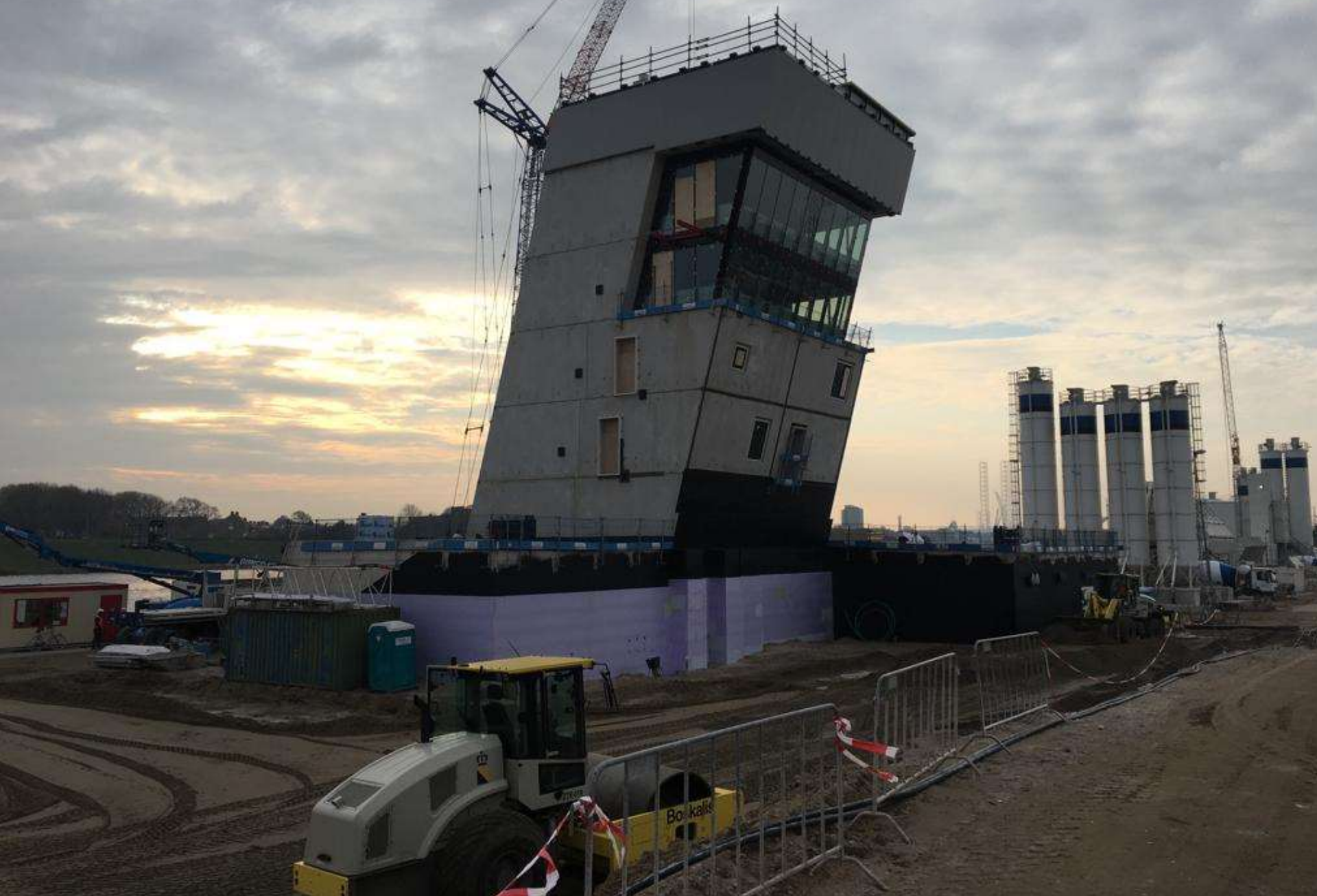
Lock operation building
