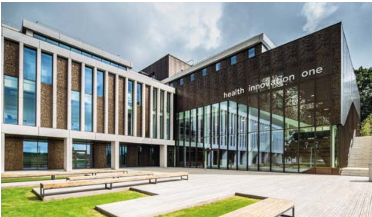
University Health Innovation Campus, Lancaster (United Kingdom) - BAM Construct UK
