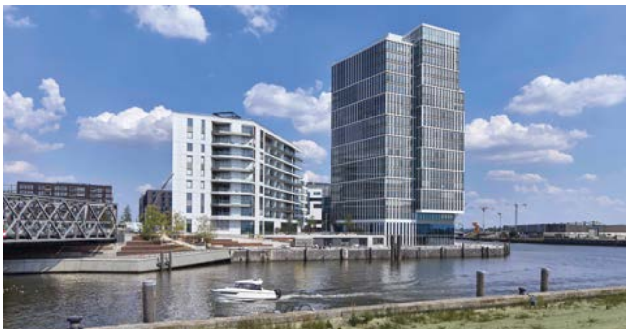
Intelligent Quarters (IQ) office and apartment complex, Hamburg (Germany) - BAM Deutschland
