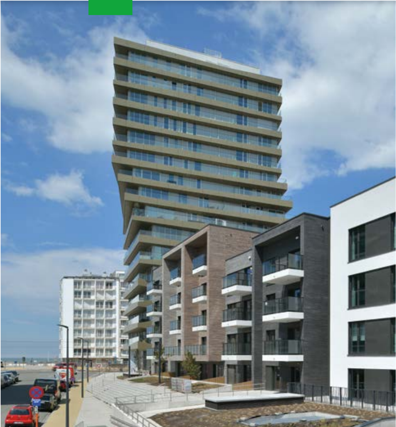
O'Sea Charme residential tower, Oostende (Belgium) - BAM Interbuild
